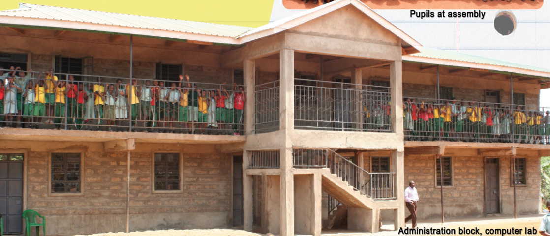
Administration block, computer lab and new classrooms
